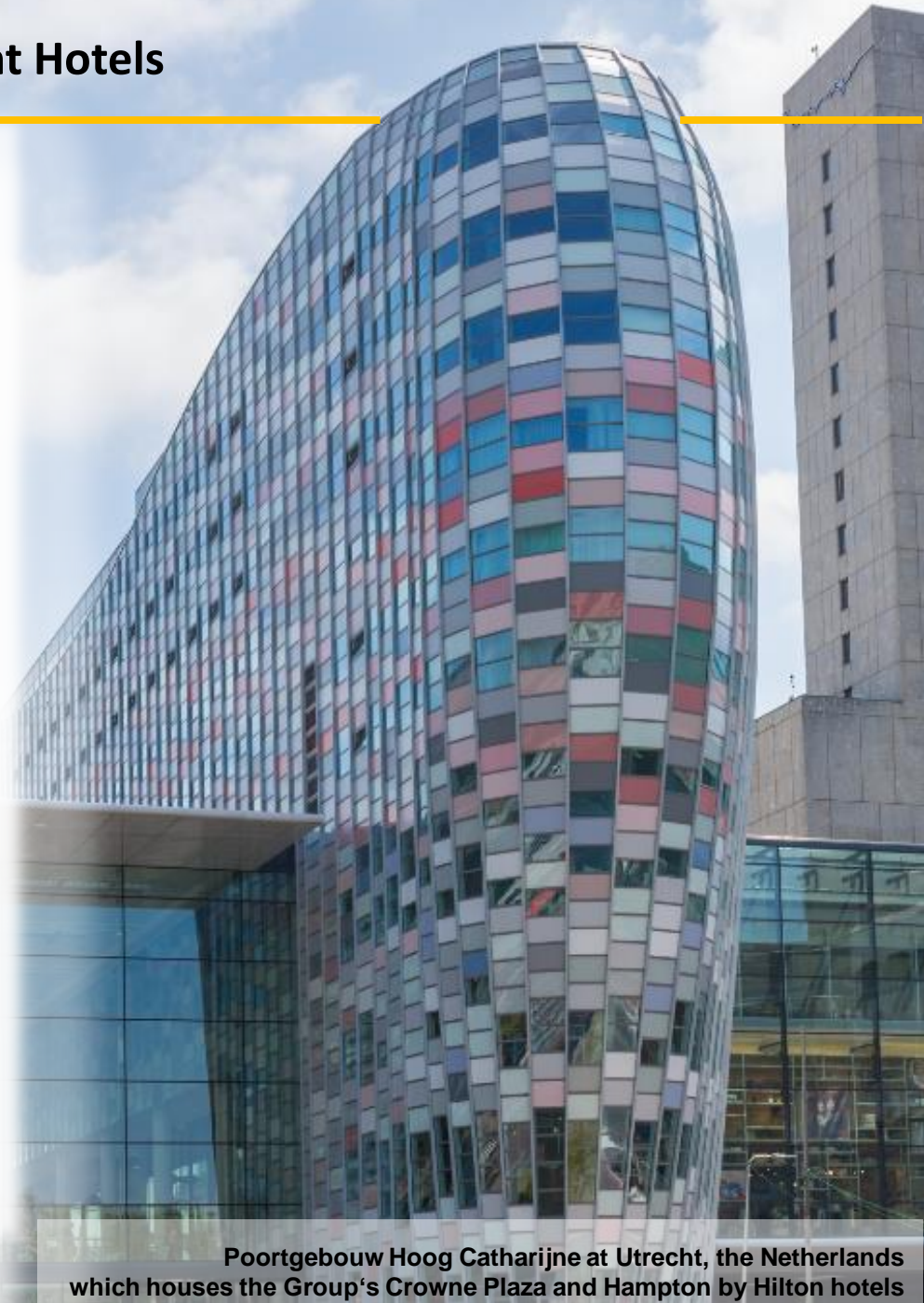
Hampton by Hilton Utrecht Central Station, the Netherlands
