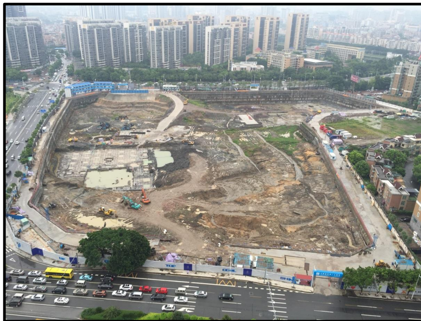
Site preparation works
