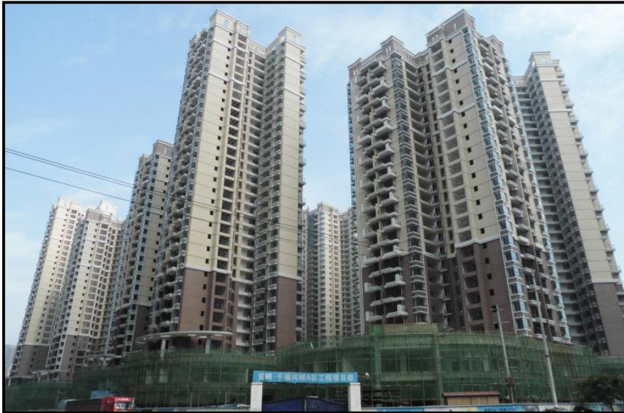
Plot A blocks under construction
