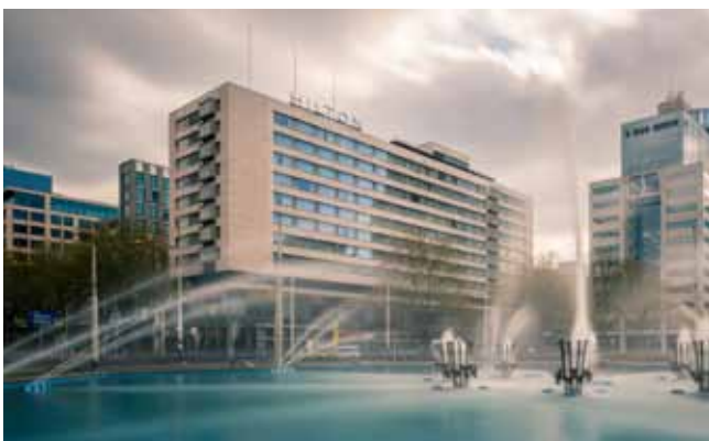
Hilton Rotterdam Hotel, Rotterdam, the Netherlands
